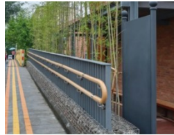
Figure 7. Installation of safety handrails
