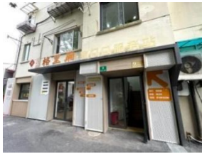
Figure 4. Gelixiang Service Station
