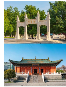
Figure 3. Front elevation shot of Dacheng Hall
